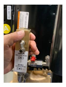
4. Disconnect the water line from the Vacuum breaker. Remove the fitting from the Vacuum breaker.
